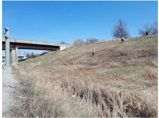
Plate 92 [E]: Previously disturbed landscaped berm and ditch within the HWY 407 ETR corridor; no potential
