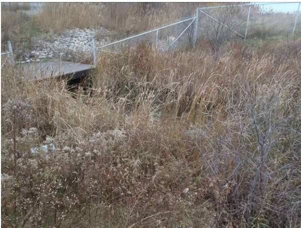
Plate 3 [N]: Culvert for Etobicoke Creek West tributary; permanently low and wet, no potential
