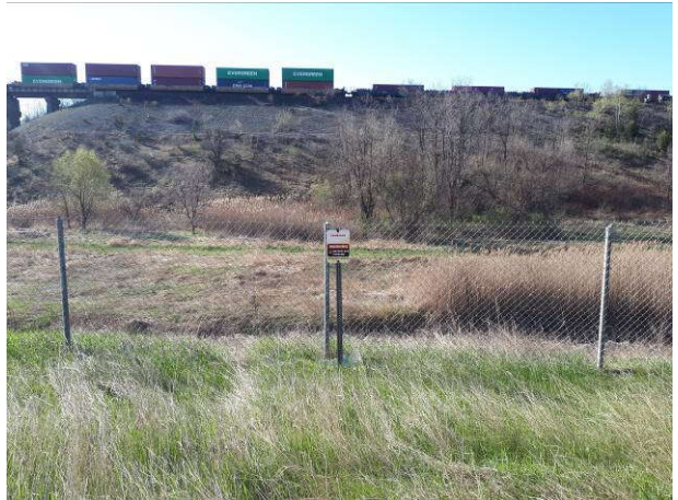
Plate 88 [SE]: Previously disturbed HWY 407 ETR corridor, redirected watercourse, and CPR raised rail bed; no potential
