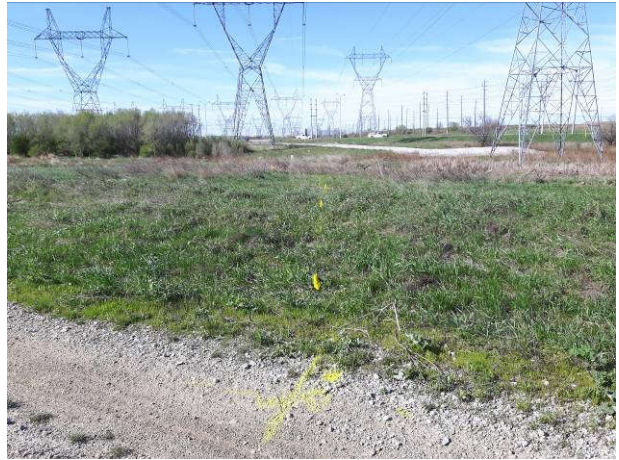
Plate 32 [SW]: Enbridge gas line subject to previous disturbance; no potential
